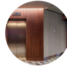
Machine Room & Shaft Access Door
