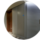
Pulley Room Access Door
